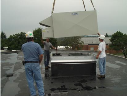
The scope of work included the installation of HVAC equipment such as heat exchangers, air separators, chemical feeders, pumps, fin tub heaters, convectors, cabinet unit heaters, horizontal unit heaters, and nine new air handling units. Our scope included both HVAC piping and sheet metal trades with the vast majority of the work being piping.
