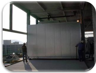
Installation included over 230,000 LBS of ductwork with large quantities containing free areas up to 30 SF. Plenums were also in excess of 15 FT x 10 FT x 3 FT. We installed over 21,000 FT of HVAC piping, numerous pieces of HVAC equipment including air handling units requiring high crane lifts for large units installed in the top floor mechanical room.
